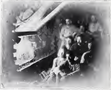
MEETING OF THE TWO SECTIONS OF THE NEW TUNNEL
